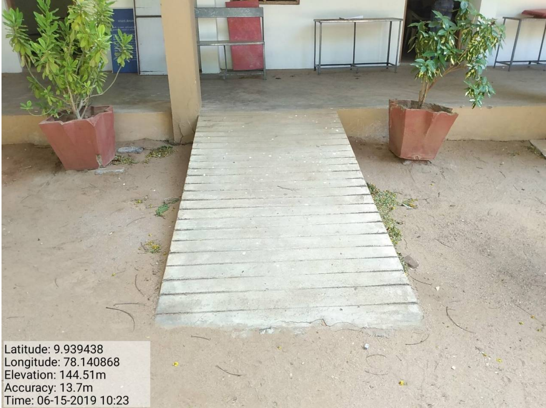
RAMP – A BLOCK
